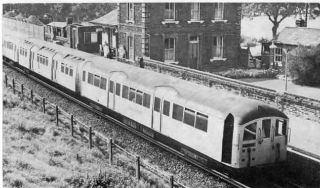
In the early 1960s, the flat-fronted shuttle units were repainted Silver to match the unpainted Aluminium 1959/62 stock on the main Central Line. This view of unit 10009-11009 at Blake Hall shows the converted 1927 Trailer (70512) which was added in 1959, and the de-icing equipment fitted to it in 1964. [R. W. Sheen]
