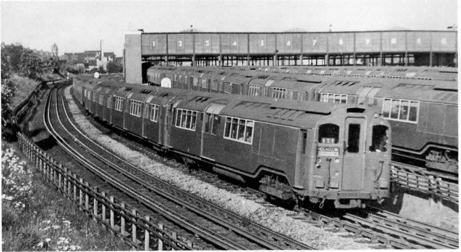
Above: A view of Northfields depot in 1949 with a seven-car Pre-1938 Tube Stock train approaching Boston Manor on a working to Hounslow West. When the Piccadilly Line first served Hounslow, both Boston Manor and South Ealing stations were non-stopped during the peaks, with the midday period, local services being provided by District trains. All off-peak Piccadilly Line trains stopped at both stations from 29th April 1935.
