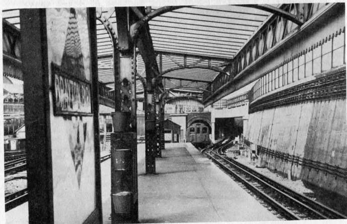
Drayton Park station on 27 March 1954 showing a Metropolitan Railway nameboard and the access ramp and track built under the uncompleted 1935-40 new works programme and subsequently connected to Highbury Vale sidings (LNER)
