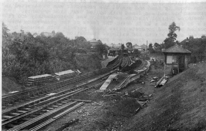
Hounslow West station undergoing reconstruction in 1926 (London Transport)
