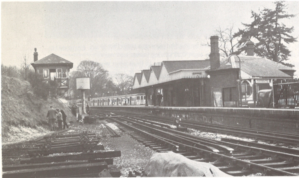
Middle Another view of Chesham station 15-4-67 showing station building, signal box and water tower.
