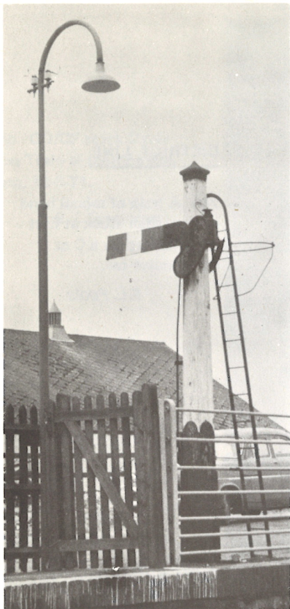
Above Three different wooden-armed, lower quadrant semaphore signals still in use at Chesham, 15-4-67.
