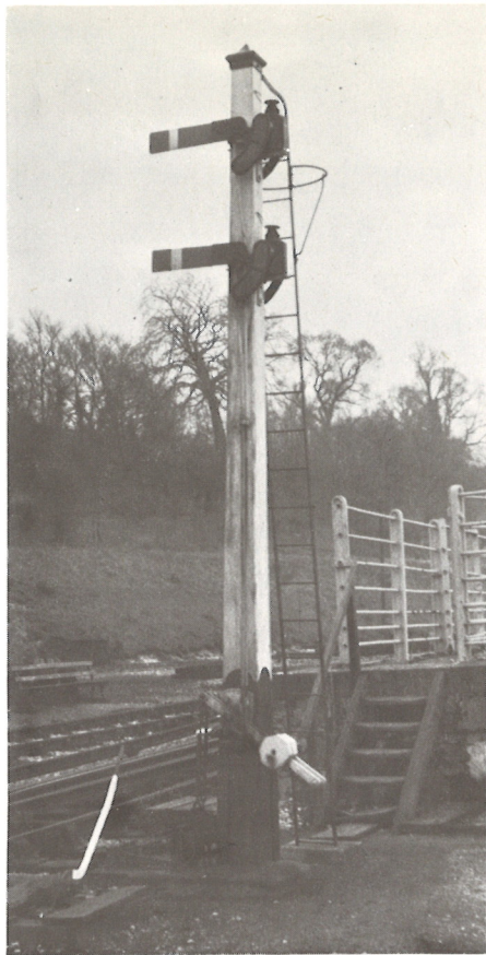
Above Three different wooden-armed, lower quadrant semaphore signals still in use at Chesham, 15-4-67.
