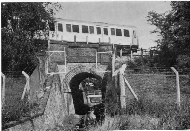
Below: Bridge U23 looking north, showing flood relief channel. The accommodation bridge, installed to give access to the working area, is visible through the arch.
