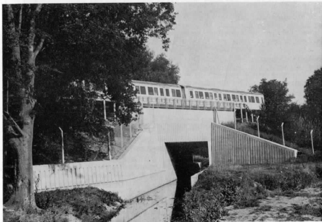
Bridge U24, as reconstructed, seen from the south side.
