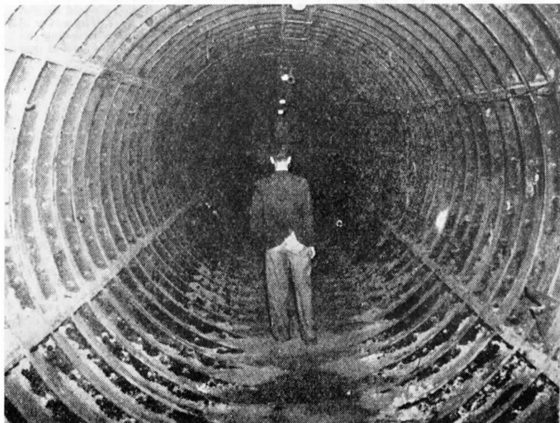
Below: View in Tunnel (since provided with flooring and seats). (Building – 2nd Aug. 1940.)
