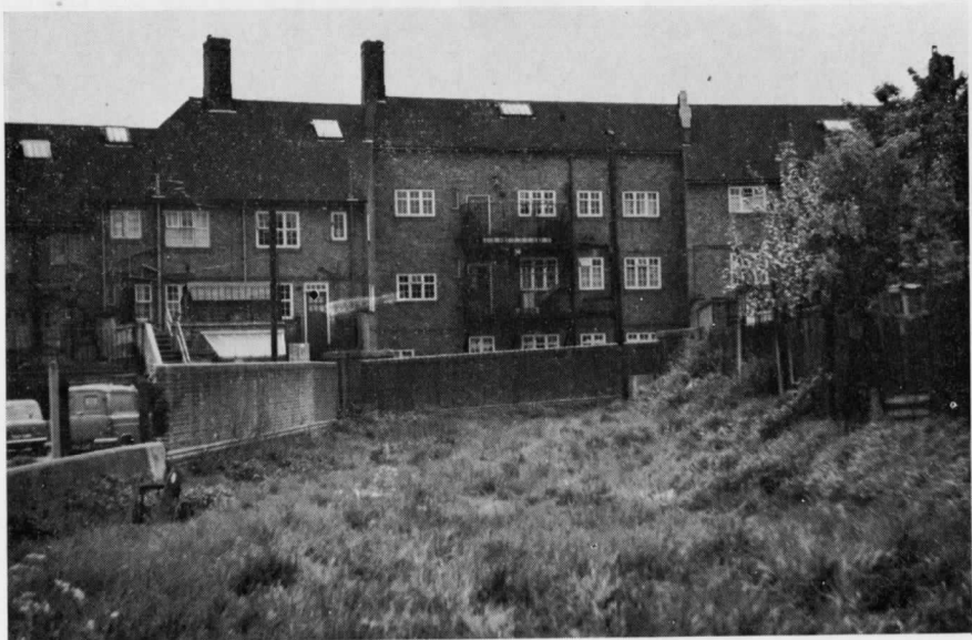
30. The site of the cutting and proposed tunnel mouth on the north side of Edgware station in May 1958. This view is largely the same today, but the rest of the route as far as Brockley Hill has since been built on. [Photomatic
