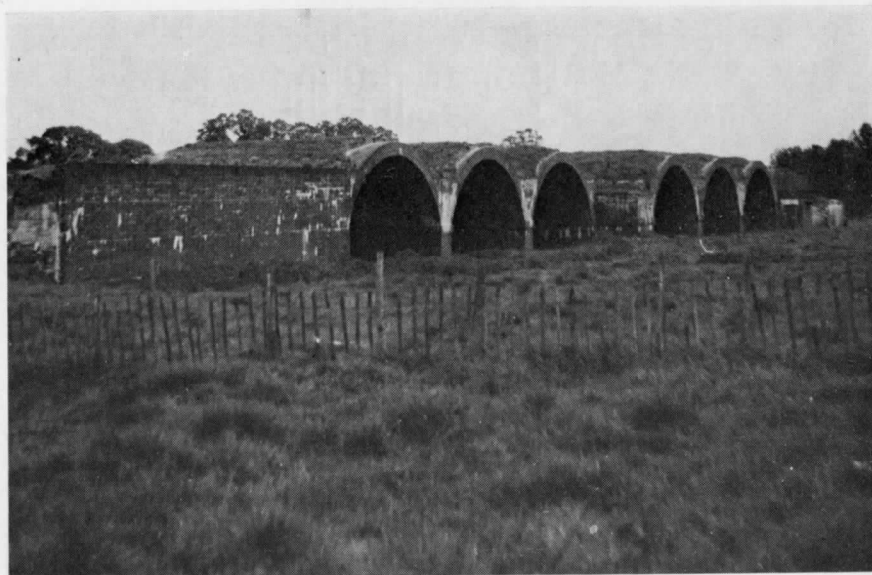
31. The brick arches of the proposed station at Brockley Hill, as they were in May 1958, having been kept in good condition right up to the time of abandonment of the extension in 1954, after which time they were allowed to take their toll from the elements. Today, just a few stumps remain. [Photomatic
