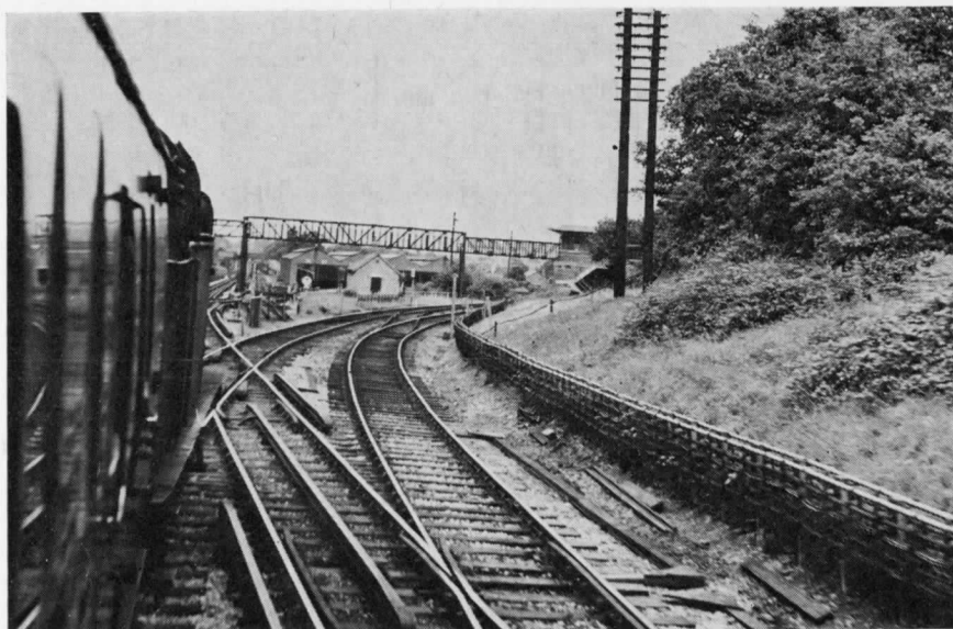
17. Park Junction, where the Alexandra Palace line diverges to the right, seen on the last day of operation on 3rd July 1954. The L.T. signal box is immediately behind the telegraph poles on the right, the former L.N.E.R. Wellington carriage shed, adapted for L.T. trains as Highgate depot, can be seen in the background.
