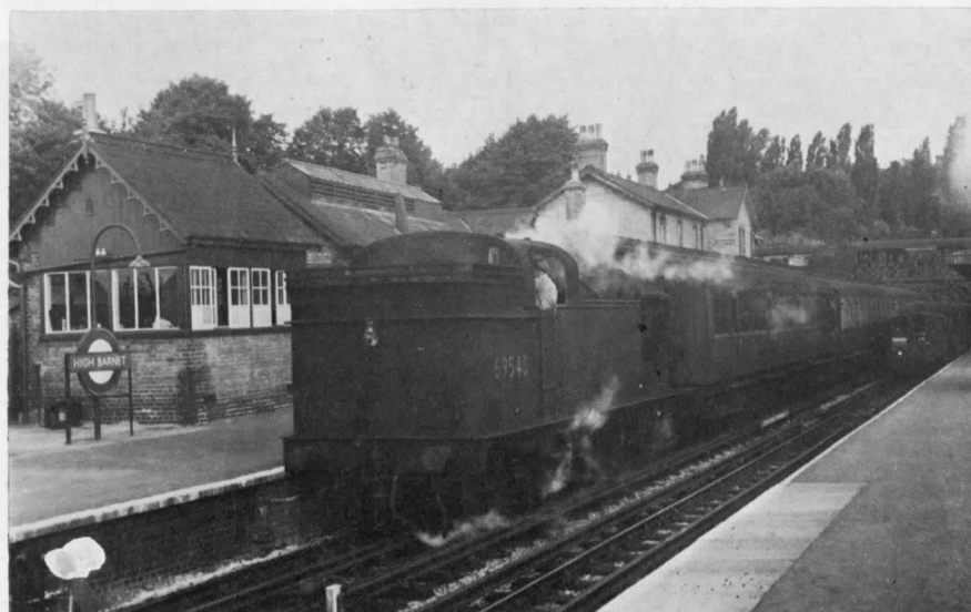
24. At High Barnet in 1956, standing next to a "short" train of 1938 tube stock, N2 0-6-2T locomotive 69540 leads a Southend excursion train. Note the old L.N.E.R. signal box. This, with others at Woodside Park and East Finchley, still stand to this day. [D. A. Jones]
