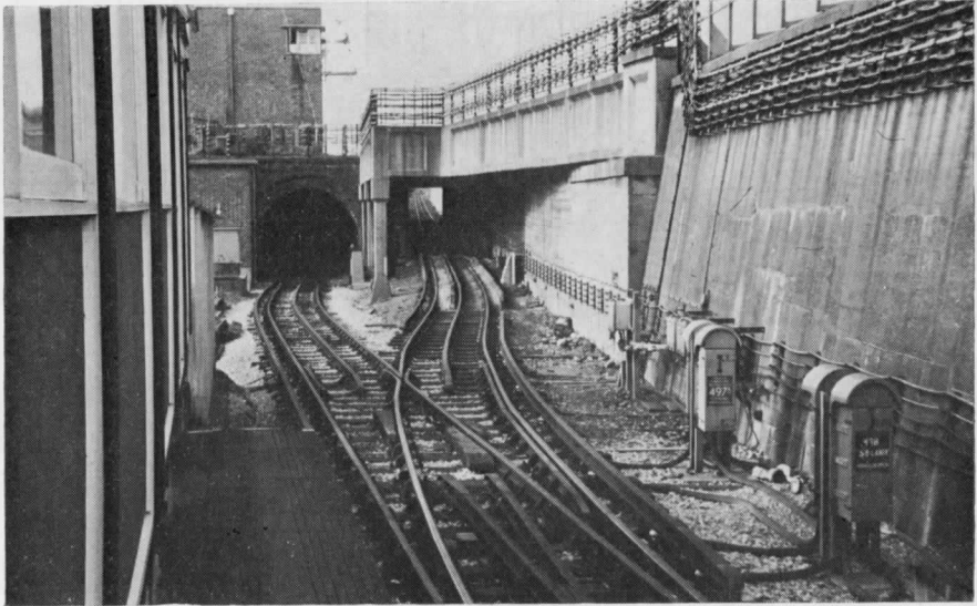
1. Drayton Park on the Northern City Line in 1969. The southbound connection, built in 1939-40 to tube gauge, and used only for stock transfers, is seen on the right. The "new" L.T. signalbox is above the G.N.&C. tunnel mouths. Note that the section switch box 497A label reads "S.B. road from L.N.E.R." as late as 1969. [James Blake]
