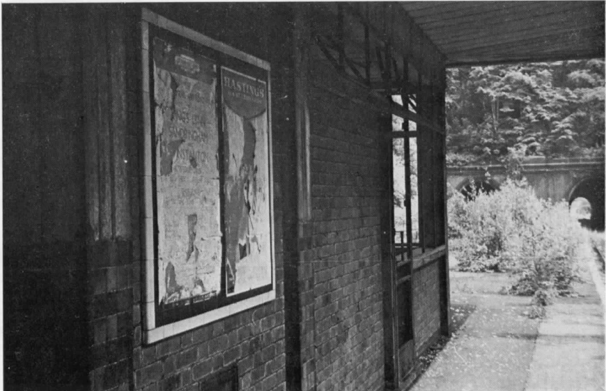
14. In 1969, fifteen years after closure, Highgate high level station was fast disappearing beneath undergrowth, as seen here. After track lifting, the trackbed too became covered with weeds, and eventually trees. This 1969 photograph shows a windowless waiting room, and also the remains of 1953 B.R. posters. [James Blake
