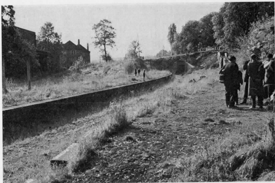
21. The site of Muswell Hill station on 17th October 1964, with the never-used substation on the left, which was demolished shortly after. Note that the bridge over the railway has been filled in, to permit the use of double-deck buses over it. The steep slope of the Muswell Hill Road can be seen in the background. [Alan A. Jackson]
