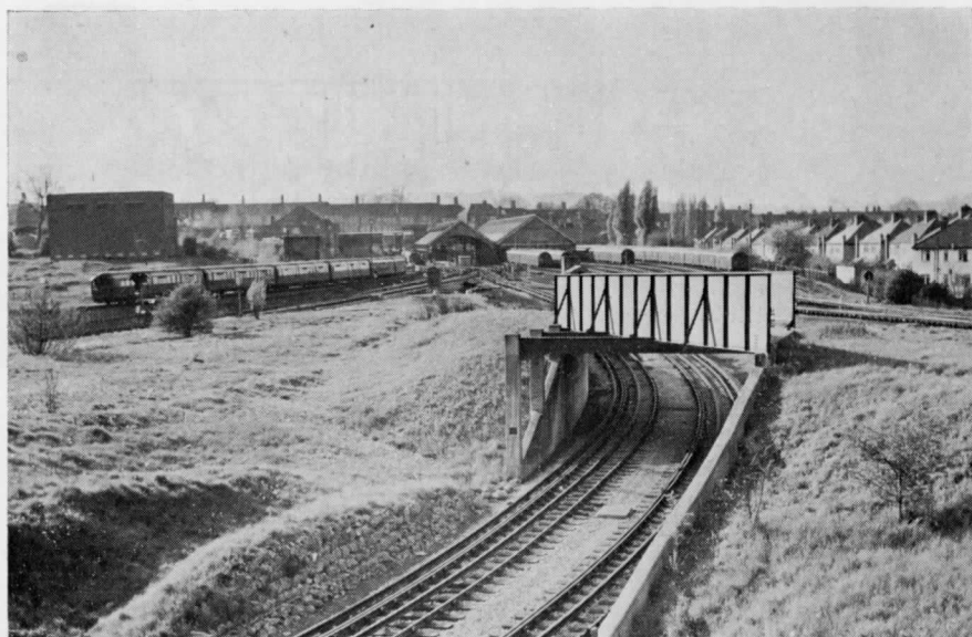
27. Looking north into Edgware L.T. station on 5th May 1956, with the flyover bridge for the northbound line from Mill Hill still in position, passing over the new route to Golders Green, which had been used only as sidings since their installation in May 1940. [Alan A. Jackson]
