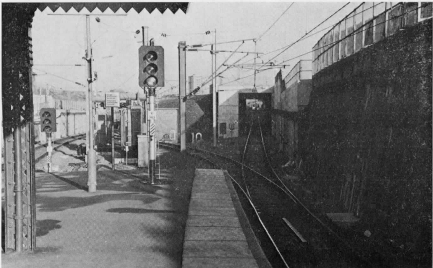
2. The same location, after takeover by British Rail. A class 313 E.M.U. approaches in the distance, using the 1939-40 ramp intended for tube trains, but enlarged to take surface gauge stock. Note that the G.N.&C. tunnel mouths have been landscaped over, and the L.T. signalbox demolished. [B. R. Hardy]
