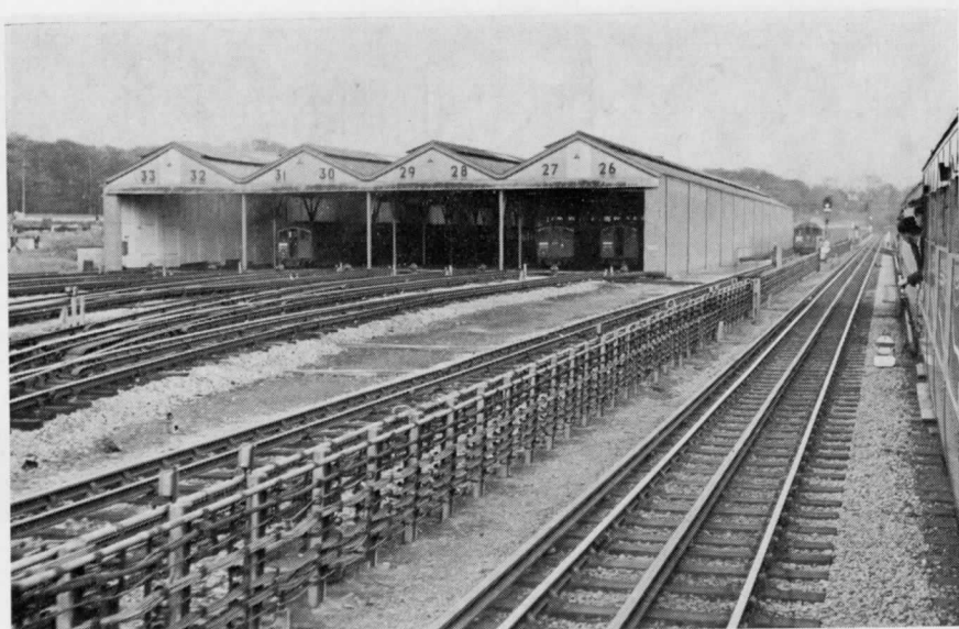
19. A view of the north end of Highgate depot, from an enthusiasts' rail tour train on 5th May 1956. When owned by the L.N.E.R., this end comprised a solid brick wall, with access only at the south end. This depot was rebuilt in 1970.
