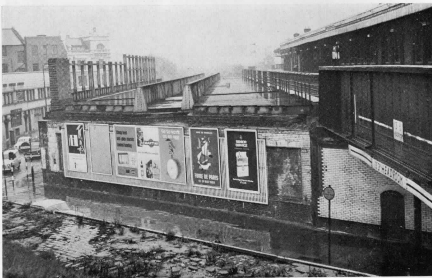
4. Finsbury Park E.R. station on 1st May 1965, showing the girder work still in position. The road in the foreground is the Stroud Green Road. The tube lines would have crossed here. [Alan A. Jackson]
