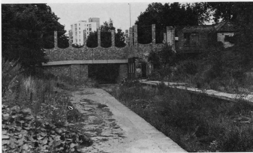
12. Having closed the line, and removed the track during 1971, steps were then taken to renew some of the bridges that forced the line's closure in the first place. A much overgrown Crouch End station platform in April 1980 shows the unusual design of the replacement bridge, the headroom and width being much less than its predecessor. [B. R. Hardy]
