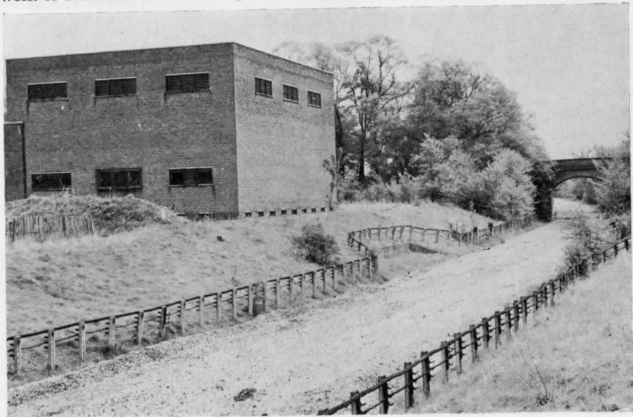
26. A view of Page Street (Mill Hill) substation on 8th May 1965, after track lifting between Mill Hill East and Edgware had taken place, but with the L.T. cabling work of 1939-40 still in almost perfect condition. [Alan A. Jackson]
