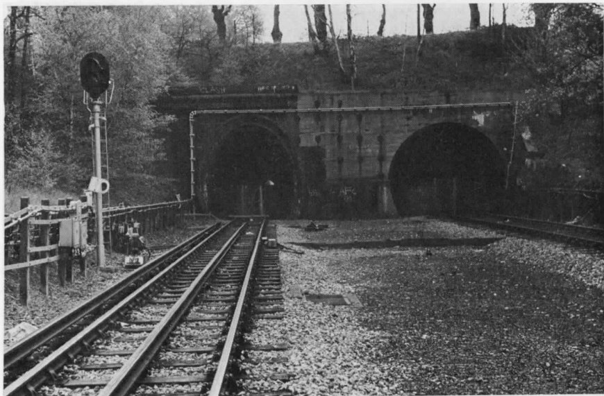
16. North of Highgate L.N.E.R. station, the line ran in twin tunnels to near Park Junction. Note that the down line tunnel mouth (on the right) has been rebuilt, having been bomb-damaged during the war. The track on the left is still used as far as the signal (now a fixed red light) by empty Northern Line trains using Highgate Wood sidings.
