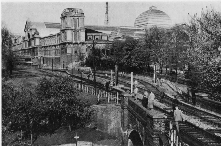
23. A view of Alexandra Palace station, and the famous Palace itself, almost two years after closure, seen on 5th May 1956. At this time, freight trains still operated on the branch, but as far as Muswell Hill only. From 8th January 1955, "no-block" working was introduced on the branch, to eliminate the need for signalmen, and trains thus had to travel at caution speed from Park Junction. [Alan A. Jackson]
