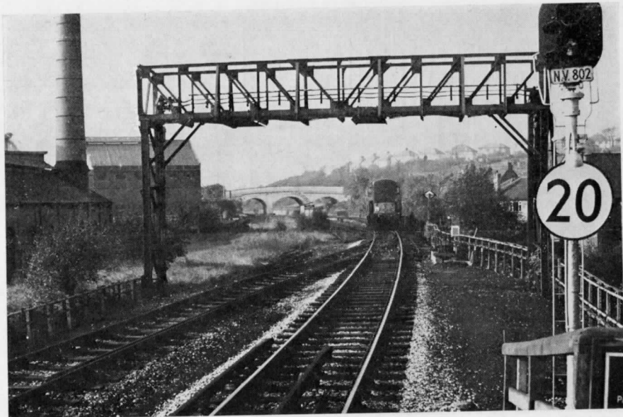
25. Looking beyond the limit of electrification at Mill Hill East towards Edgware on 13th November 1962, with B.T.H. Type 1 800hp Bo-Bo diesel locomotive D8242 shunting on a freight working. These locomotives were fitted with tripcocks for operating on L.T. sections of line. By this time, all the goods yards up to High Barnet had been closed, the only goods trips scheduled being to Mill Hill and Edgware, albeit only until early 1964. [J. C. Gillham]
