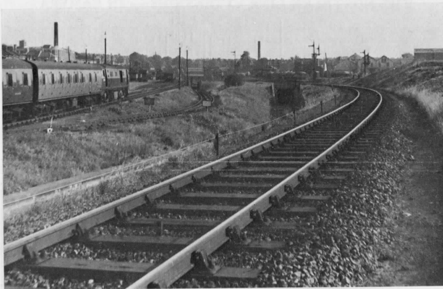
3. North of Drayton Park in the early 1960s, the southbound ramp can be seen just to the right of the diesel-hauled Broad Street train, descending to Drayton Park station. The almost completed but never connected northbound ramp can be seen to the right of that. This was finally put into use in 1976 by B.R., having stood wasted for over 35 years. The line in the foreground is the "down" line from Broad Street, which crosses over the proposed tube lines. [L.U.R.S.]
