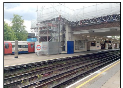
Opposite: (Lower) Work began on 19 April 2021 on the repair of the concrete canopies at East Finchley station, which was expected to continue through to the end of June 2021. Scaffolding was erected to enable access to the canopies to enable the breaking out and repairing of the defective areas of concrete. Most of the actual work was scheduled to be done during daytime hours.
