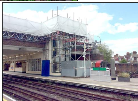
Opposite: (Lower) Work began on 19 April 2021 on the repair of the concrete canopies at East Finchley station, which was expected to continue through to the end of June 2021. Scaffolding was erected to enable access to the canopies to enable the breaking out and repairing of the defective areas of concrete. Most of the actual work was scheduled to be done during daytime hours.
