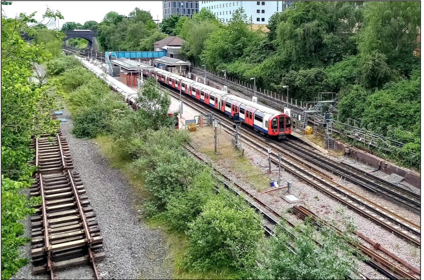
Above: North Acton on 6 June 2021 with a westbound train of 1992 Tube Stock awaiting departure. Note on the left the lifting of the main line track from the junction of Old Oak Common.
