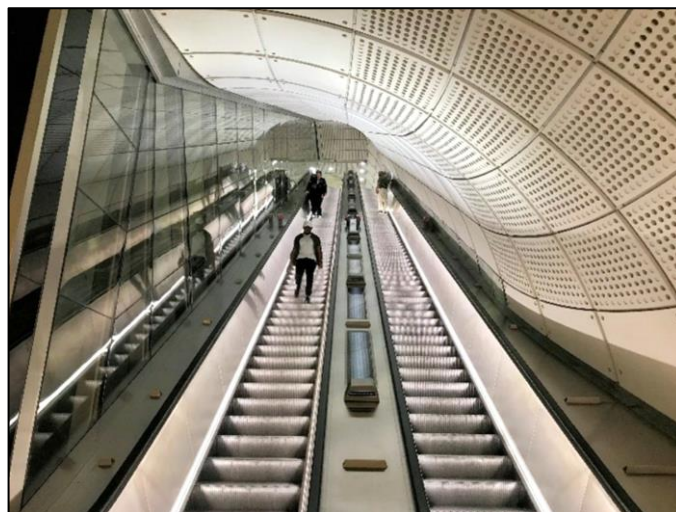
A second set of escalators is required to reach the platforms from the Interchange Level (east). These are escalators Nos. 10 & 11, plus Lift No.8, whose glazed shaft is on the left.
