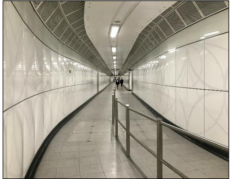
A long corridor links the Bakerloo Line platform concourse at Paddington LU with the Elizabeth Line station. This is the view looking towards the latter. The tiling pattern is inspired by Brunel's 1854 train shed roof.
