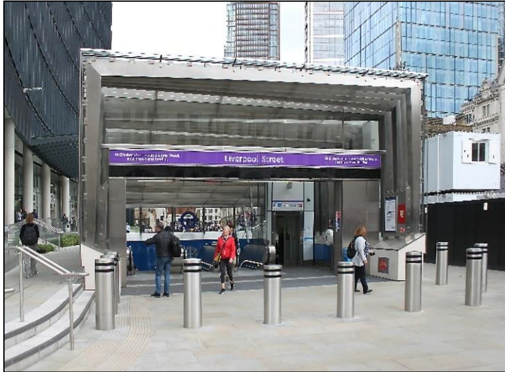
Liverpool Street's Eastern Entrance in Broadgate. Visible are escalators Nos. 12, 11 & 10, and inclined Lift No. 9.
