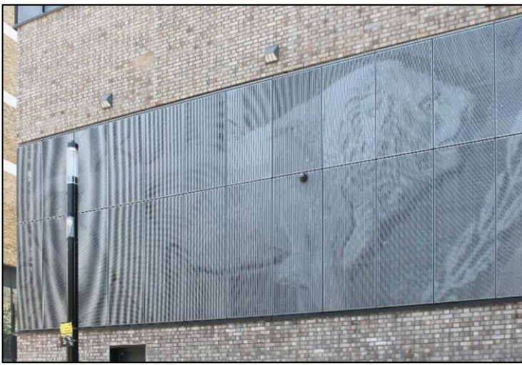
Part of the exterior bronze panelling bearing an image from WW1 Memorial Death Plaques.
