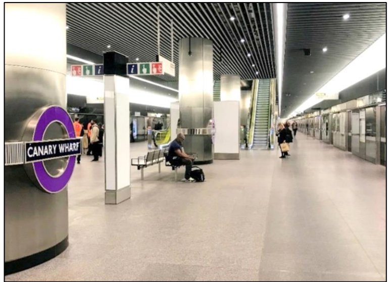
This is platform level at Canary Wharf looking west. The oval support columns are clad in stainless-steel and a slatted ceiling helps to hide services and utilities.
