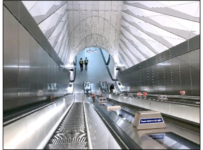
Escalators Nos. 24, 23 & 22 at Moorgate between Moorfields ticket hall and the mezzanine level (west).
