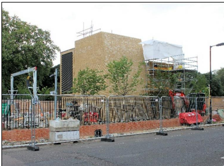
Above: Kennington Park ventilation shaft on the southbound line.
