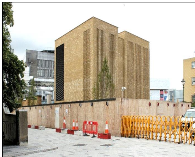
Above: Kennington Green ventilation shaft on the northbound line.
