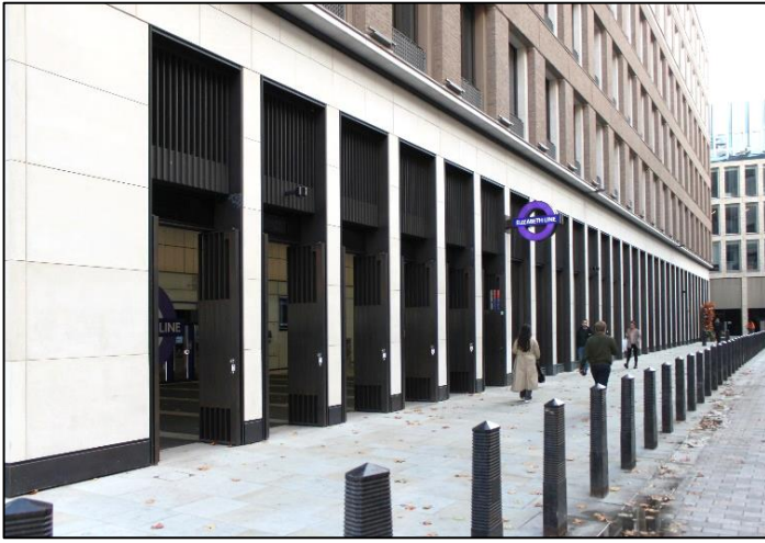
Above: Hanover Square entrance is open on two sides. This is the north elevation, with the bronze doors seen in the open position.
