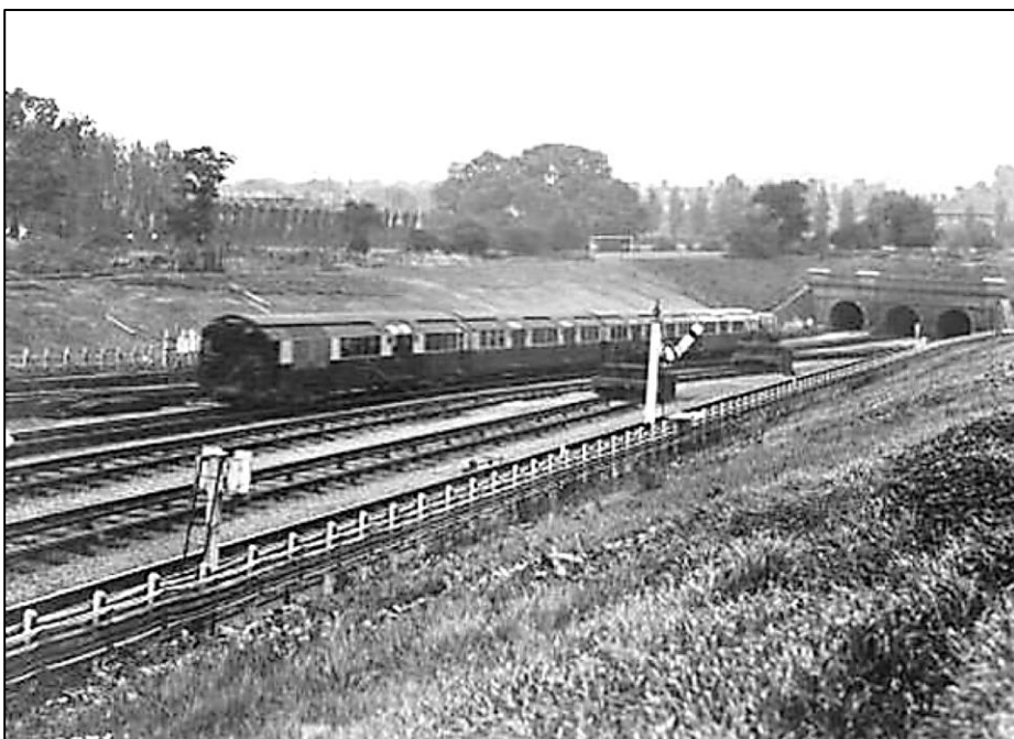
Figure 8: A 4-car train of new 1923 Tube Stock approaching Golders Green after the completion of track alterations for the extension to Hendon. The outer home signal is an upper quadrant semaphore. Nearer to the camera is a pair of 2-aspect fog signals for the inner home junction signal. Photo: LT Museum.
