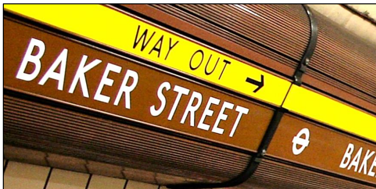
Left: A Bakerloo Line platform frieze and Cable Management System at Baker Street as installed circa-1979. The lettered areas have since been covered with more modern signage.
