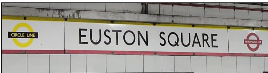
Left: Euston Square has the last surviving full set of original 1950s/60s enamel platform friezes. Separate roundel types were needed on sections of the sub-surface railway where two lines served the same platform. The Circle Line version carried a black bar to aid legibility.
