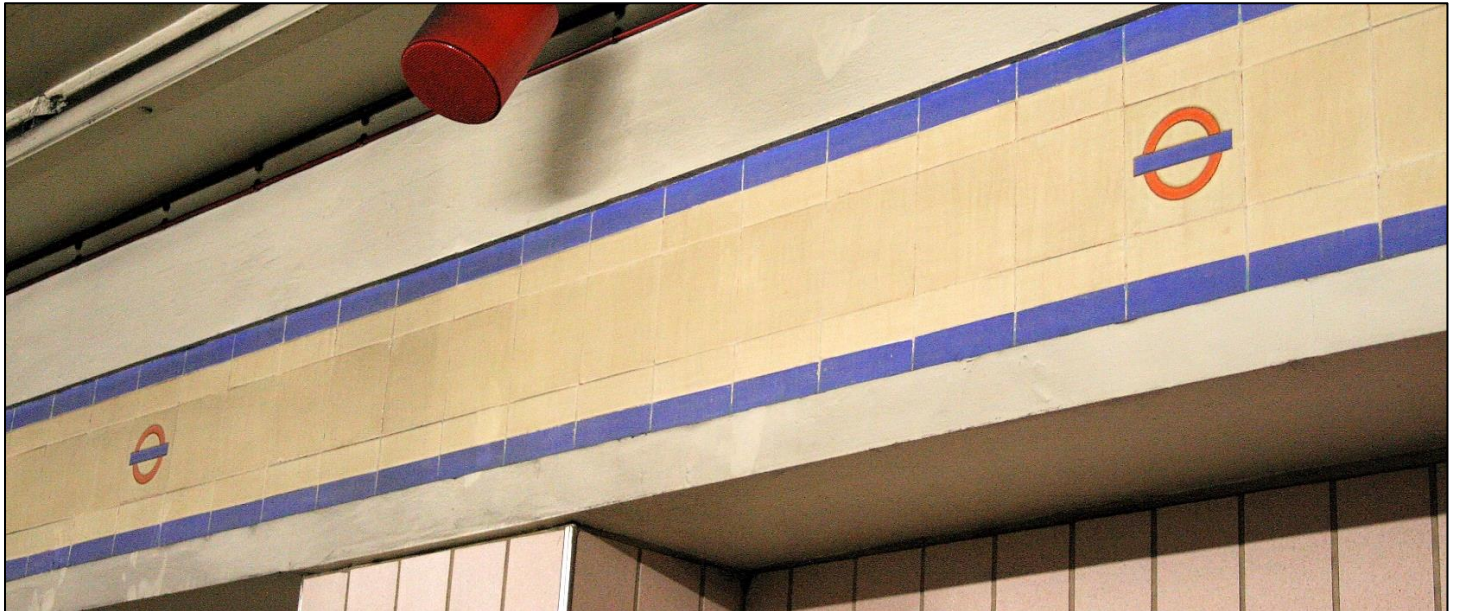
Above: The unfinished 1947 platform frieze at Redbridge. Although most of the station was given new light pink tiling in the 1980s, the frieze area was left untouched and shows the blue relief colour originally chosen for this location.
