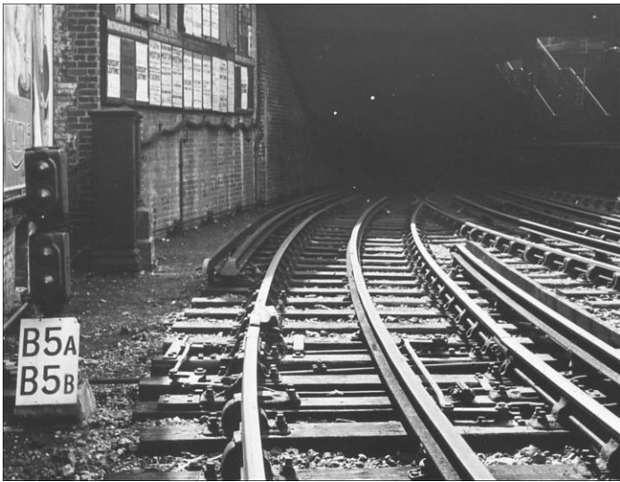
Figure 2: A derailer on the exit of No.6 Siding at Edgware Road, Metropolitan Railway, after the completion of the station rebuilding and resignalling in 1926. It can be seen on the left hand running rail. It was operated by its own lever in the signal box. Your author was familiar with this device as it was still in place in the 1970s, even though the area was resignalled in 1951. At that time, the siding became known as No.26 Road and the Signal B5 A became OP10 and was replaced by a disc shunt signal. The derailer worked by lifting the wheel flange up over the running rail, dumping the wheel into the ballast, effectively stopping the train. Interestingly, signal B5 B seen here was not used but it was installed in anticipation of the proposed loop line to Willesden Green. The derailleurs were finally removed in 2010. Photo: Westinghouse Archive & Chippenham Museum.
