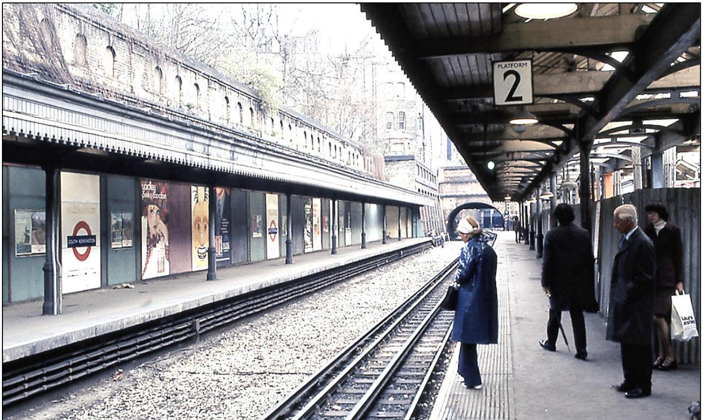
Above: South Kensington in 1973 looking east along eastbound District Line platform 2. On the left, the disused inner rail Circle Line (ex-Metropolitan Railway) platform 1, which had closed on 8 January 1967, with its 1906-07 canopy and valancing and 'panel' roundel signs remaining. Above the canopy is part of the original 1868 brickwork. To the right, the former bay road area and later the station garden is screened off to allow work on providing stairs and a subway to new escalators 1, 2 & 3. Platform 2 had originally been the outer rail Circle Line (ex-Metropolitan Railway) prior to the current arrangements being introduced. The platform area nearest the white line has now been given an early form of non-slip surface.
