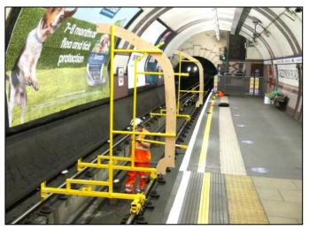
**Left**: The 2024 Tube Stock train profile jig in use at Caledonian Road in late-June 2021.
