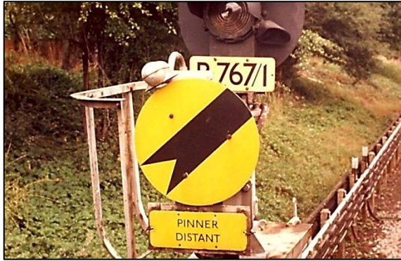
Figure 3: A disc distant signal provided on some lines where main line freight trains operated over the same tracks as Underground trains. This one is on the Metropolitan Line and, to clear, it required A761, A763A, A763B and A767 all clear (the Pinner starter, homes and the next intermediate signal to be off). Note that these signals were not numbered but they were named. They were often mounted on existing Underground signal posts. Photo: LURS Collection.
