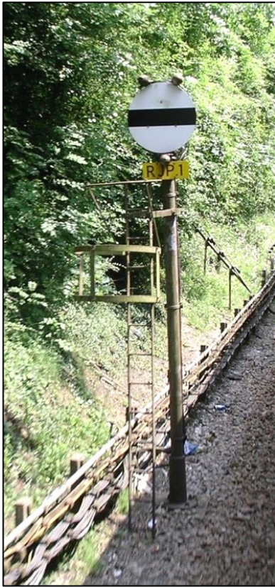
Figure 5: To give main line trains adequate warning of the position of the home and starting signals at Rickmansworth SB, two e.p. operated banner repeater signals were installed on the approach to the station. They replaced two yellow band mechanical banner signals. The new signals were externally illuminated discs, like shunt signals but with a black band on a white ground instead of a red band. The first was for the home signal given a standard Underground repeater number (RJP1, see here in the 'on' position), the second was RJP2 for the starter. Photo: B.R. Hardy.
