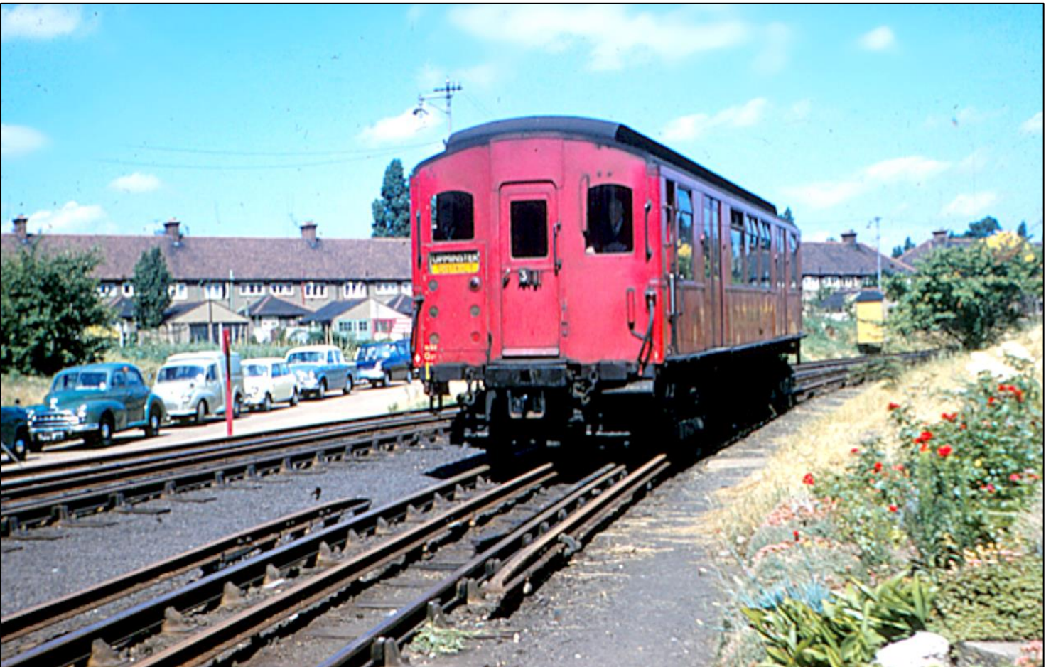
Previous Page: (Centre, Left) Acton Works also had high-level 'Alps' sidings, where a Metropolitan electric locomotive and brake van (B552 of 1890 Metropolitan Railway vintage) are seen beside an R38 driving motor car.
