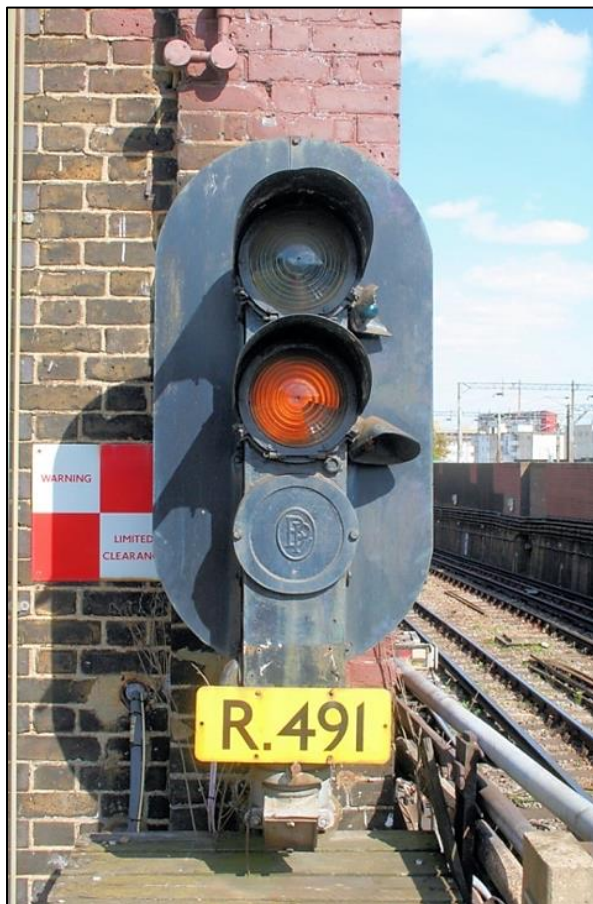
Figure 4: A 2-aspect repeater signal at Queen's Park that has been recycled from a Metropolitan Railway 3-aspect signal. The bottom aspect has been blanked off by a plate lettered BP. BP was the British Power Railway Signal Co., who supplied some signals and signal frames for the Metropolitan Railway. Note the rusted condition of the upper of the two 'pigs ears' to the side of the main lens. This signal dates from the 1925-32 period. Photo: Kim Rennie.
