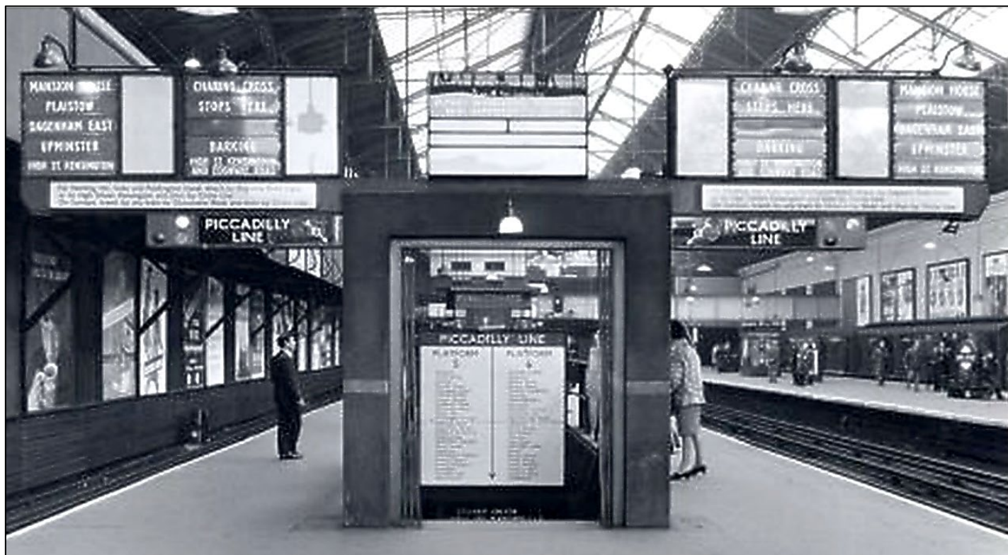
Above: Earl's Court in the 1960s with the indicators now using Condensed Johnston. These plates remained in use until 2007. Note that a 'switchable sign' has now been fitted above the stairs.
