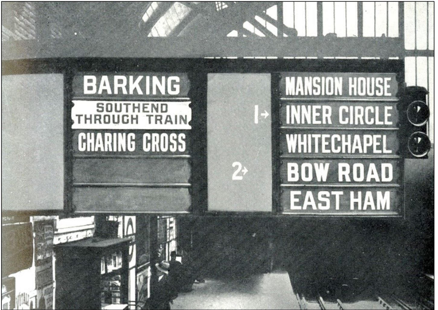
Above: A two-panel 10-plate '1,2,3' eastbound indicator. The SOUTHEND THROUGH TRAIN plate suggests this is 1910 or later. The arrows adjoining the numerals were omitted on some signs. Note the 'coffee pot' platform repeater on the right, some of which remain in use today.
