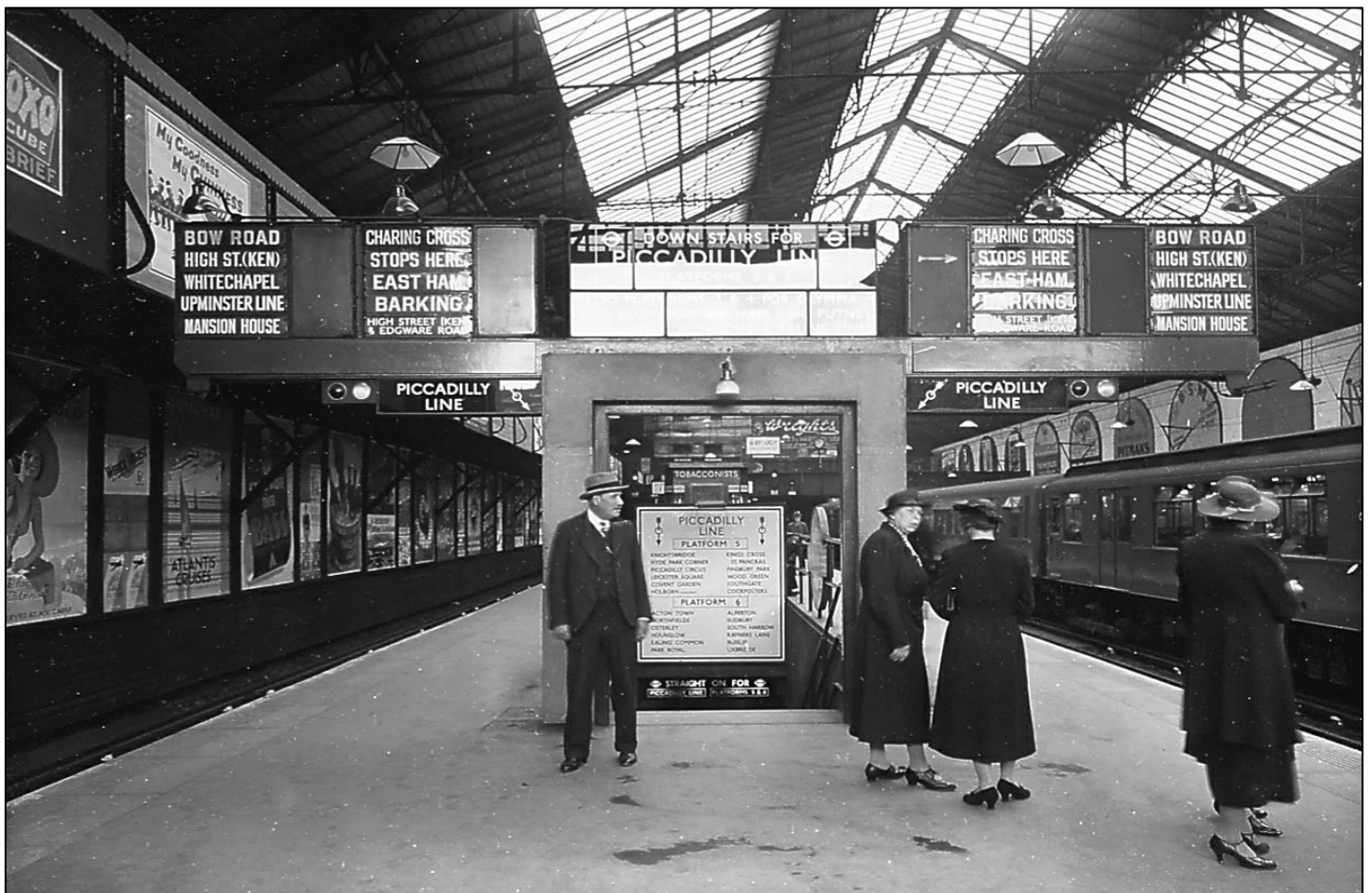
Above: By 1939 the indicators had become aligned with each other and were mounted on concrete beams above the stairs to the Piccadilly Line escalators. The stairs also gave direct access to the 1937 Exhibition Subway. Note the spot lamps added later to illuminate the plates.
