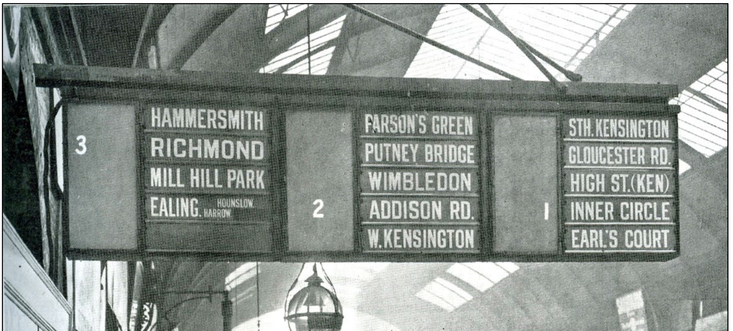
Above: A three-panel 15-plate '1,2,3' westbound indicator at St. James's Park (also illustrated in Underground News No.733, page 36). The various branches of the MDR meant more destination plates were required in this direction. The EALING plate has HARROW and HOUNSLOW in smaller letters as some trains divided at Mill Hill Park. The UXBRIDGE name has been covered up as the MDR was not serving this line at the time.
