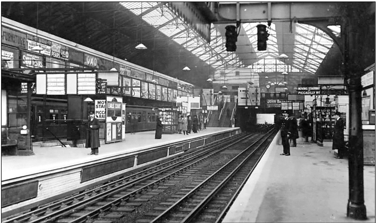
Above: A view from platform 3 looking east. Stairs lead down off the platforms and the 1911 escalators are probably now in place. The eastbound indicator was suspended then from a triangular bracket.
