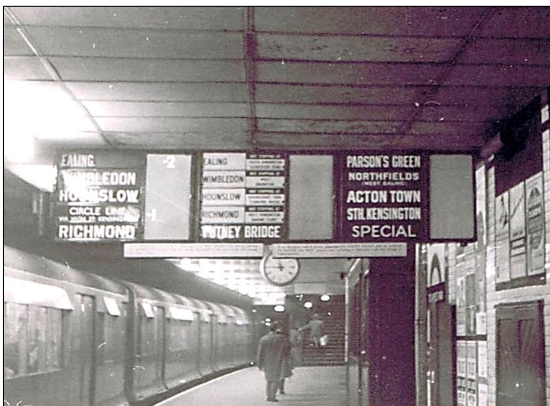
Above: The same indicator at St. James's Park in 1964 after the station was rebuilt as part of the 55 Broadway complex. NORTHFIELDS (WEST EALING) and HOUNSLOW have changed places, whilst INNER CIRCLE had been replaced by CIRCLE LINE via HIGH ST. KENSINGTON in Johnston. GLOUCESTER ROAD is now SPECIAL and appears in Johnston and the NON-STOP/NOT STOPPING AT plates have been modernised and are coloured black-on-yellow.
