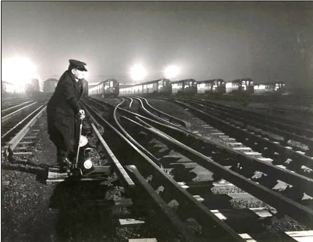
Figure 7: A posed photo of a Ground Shunter setting up a road in Northfields Depot (Boston end) on a cold day in March 1955. With a full depot, it is probably early in the morning, but shunters didn't have to set up roads for trains leaving the depot because the points from each road were trailing, hence the conclusion that the photo is posed. Trains were called down to the exit signal through a loudspeaker system. The shunter has his handlamp with him that he will use to signal to drivers when necessary. In the yard there are Piccadilly Line Pre-1938 (Standard) Stock, 1938 Tube Stock and District stock. Photo: LT Museum.
