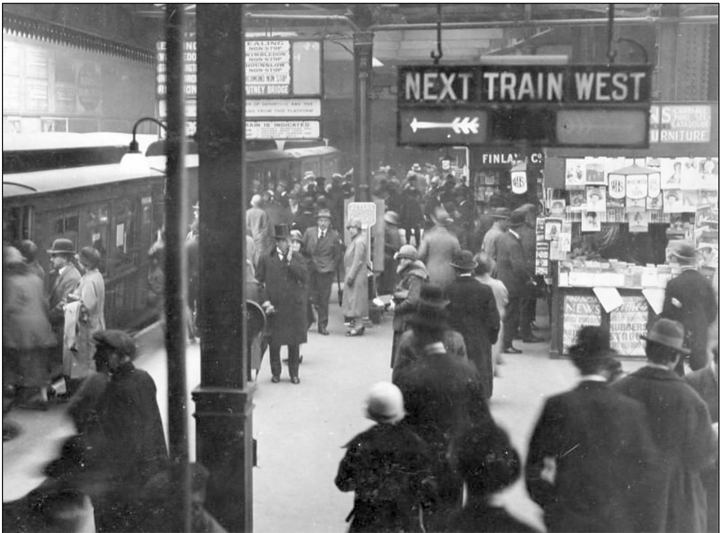
Mansion House platform 4 (now 1) looking west in 1924, with the hanging 'First Train Out' indicator to the fore. The westbound indicator had fixed "When No Through Train is Shown ..." signage below it.
