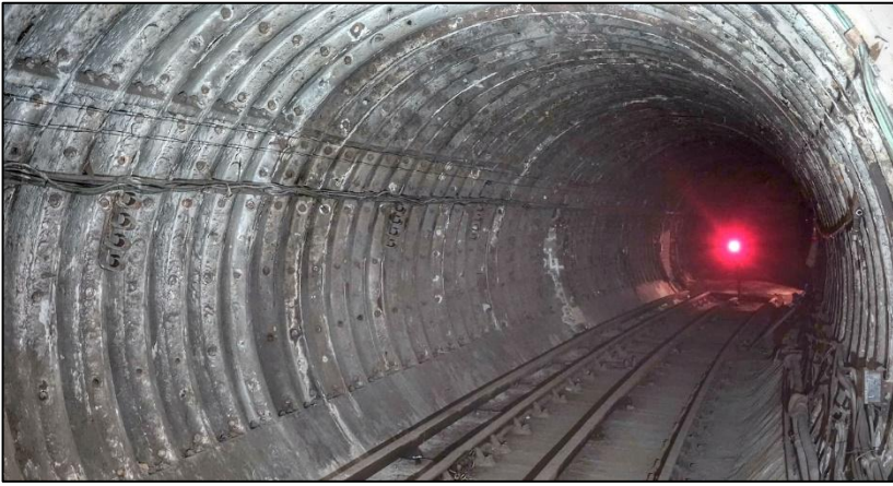
Left: The end of the line in the overrun tunnel with the fixed red light illuminated.
