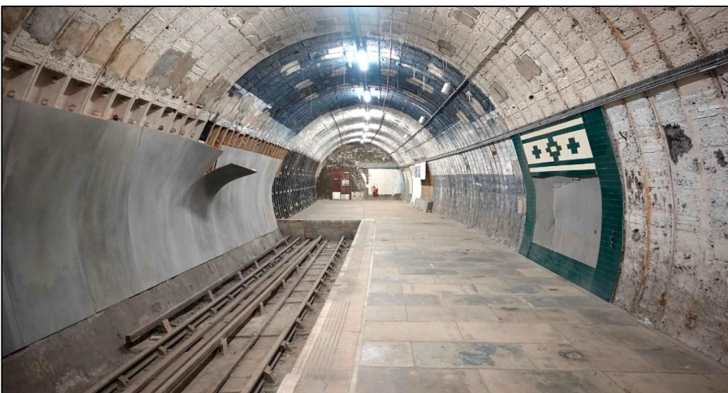
Overleaf: (Top) In the opposite direction and looking towards the end of the line, showing that more of the original tiling remains. The way in/out is left of centre with stairs leading up to the passageway and crossing the track (see above). Note the open door in the centre of the photograph, which leads to the incomplete subways to the back of the lifts.
