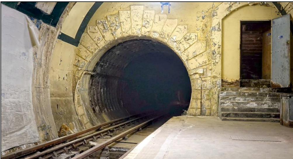
Left: On what was the operational platform until the line closed on 30 September 1994, this looks to the overrun tunnel, in which one of the two cars was uncoupled and stabled during slack hours pre-WW2. On the right is the unfinished access to the back of the lifts, which was never opened. The condition of the voussoir (around the tunnel mouth) leaves a lot to be desired.
