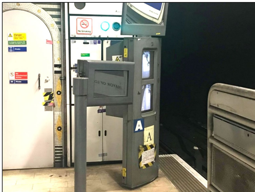
Figure 6 Top: A photo of the blank dwell time indicator screen at Finsbury Park WB on the Piccadilly Line next to the platform OPO monitors. The system was tried for a time in 2012 but quickly fell into disuse. Photo: LURS Collection.
