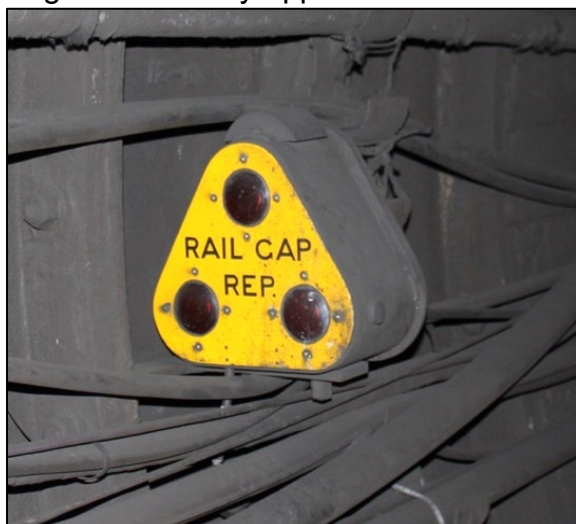
Figure 2: A Rail Gap Repeater at Stockwell. When lit, it uses three yellow lights to show that the RGI ahead is lit. Repeaters are only provided where the sighting distance for the RGI itself is not sufficient to provide enough stopping distance. Photo: Kim Rennie.
