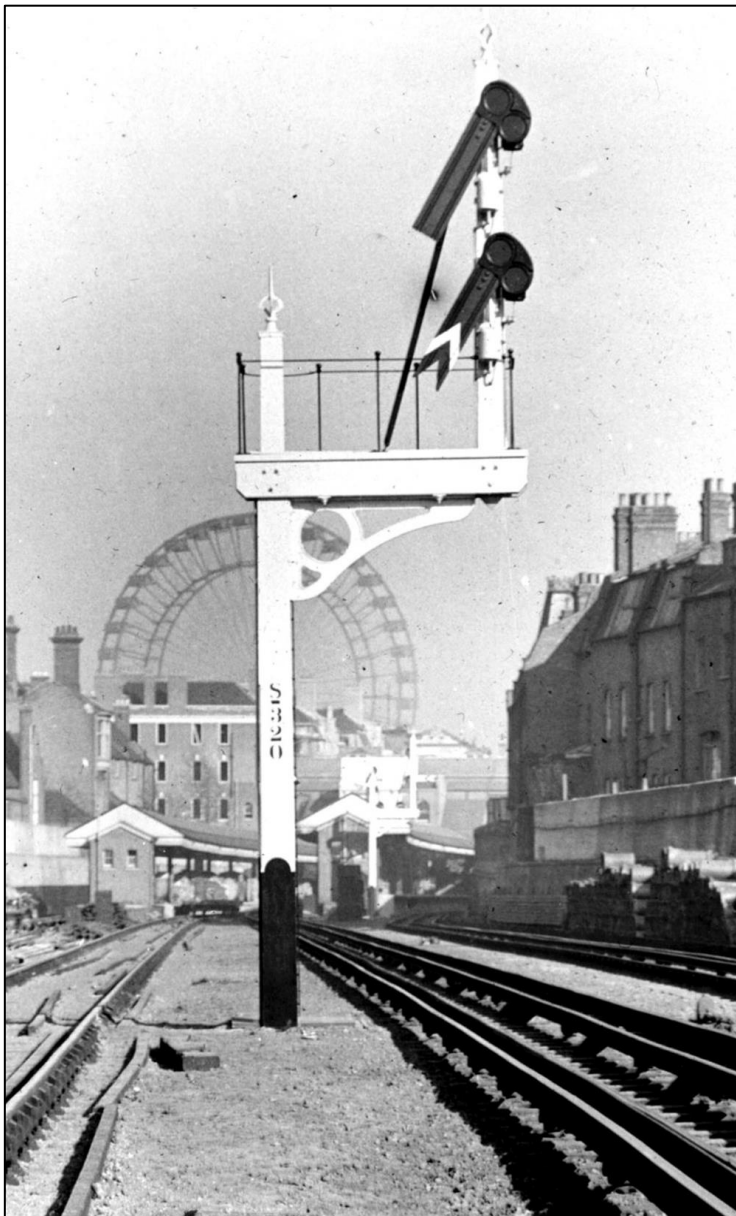
Figure 3: A new automatic home signal with an automatic distant on the approach to Barons Court eastbound District road. Both signals were painted red, with the usual fishtail on the distant signal. Both signals showed red and green aspects at night, in accordance with the convention of the time. The trainstop for the stop signal can just be seen to the right of the track. The date of the photo is believed to be 1905. The Piccadilly Line tracks can be seen under construction on the left hand side. At the time, the District had the two southern tracks and the Piccadilly Line was to use the new tracks on the left to give them access to the existing terminal platforms at Hammersmith. In the background, the big wheel of the Earl's Court exhibition site can be seen. The use of a distant signal here was a special requirement because of the operation of Midland Railway freight trains to the coal yard at West Kensington. It was not required by District trains, which would normally stop at Barons Court but the heavy and largely unbraked coal trains required early indication of the starter because of their poor braking capability. The District did not use repeater signals until shortly after this signal was installed. Photo: Courtesy Westinghouse Archive & Chippenham Museum.
