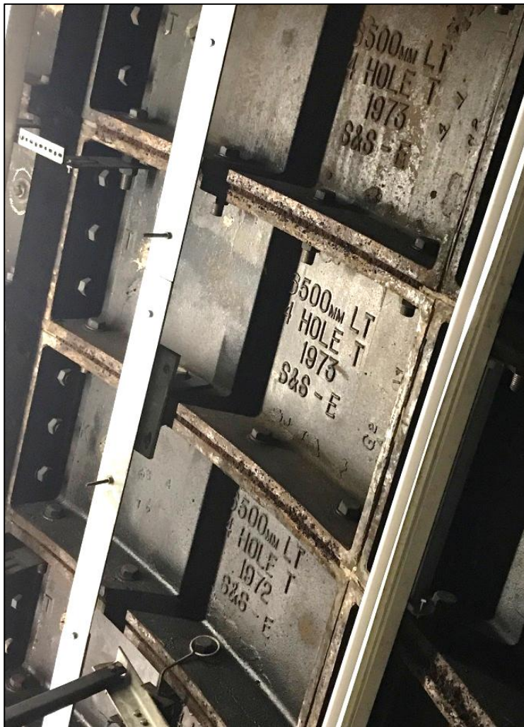
Above: Platform 4 tunnel segments by Stanton & Staveley.
