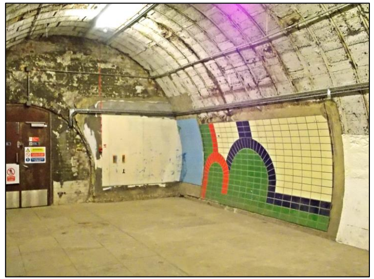
Above: The east end of the 1910 disused platform looking east. The tunnel access towards Holborn is now sealed, as can be seen.
