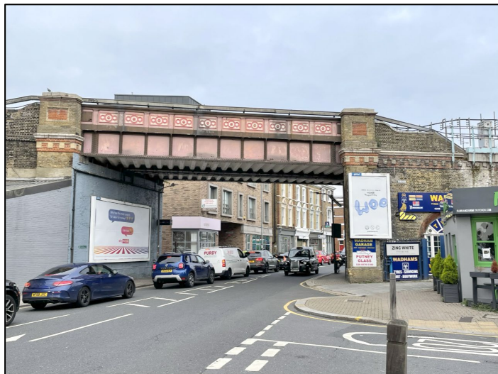
D223 Putney Bridge Road (east side).
