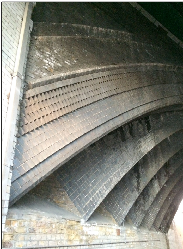
Above: MR12 Iverson Road skew arch detail.
