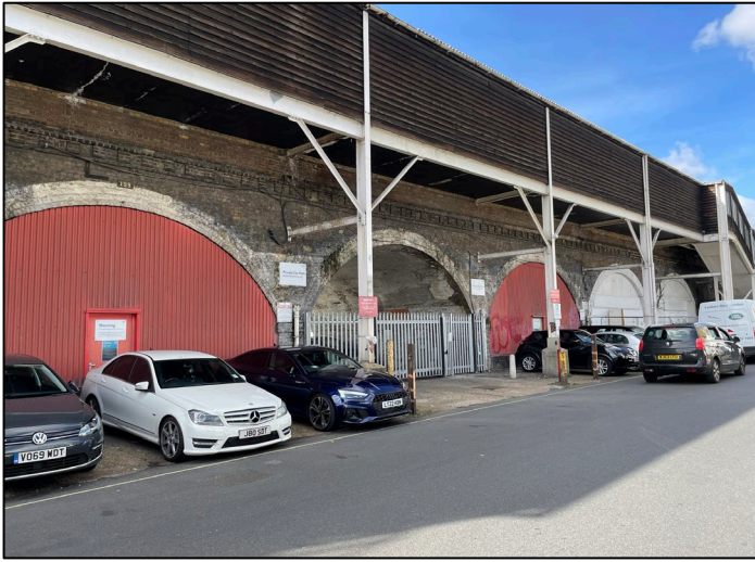
HC22 viaduct with Goldhawk Road platforms.
