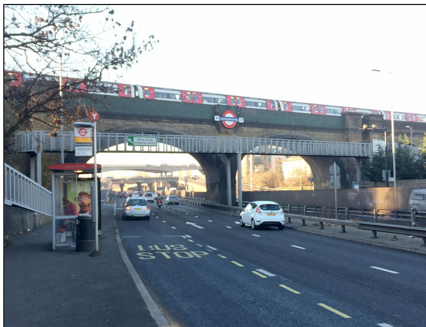
Above: NT16 A406 viaduct.
