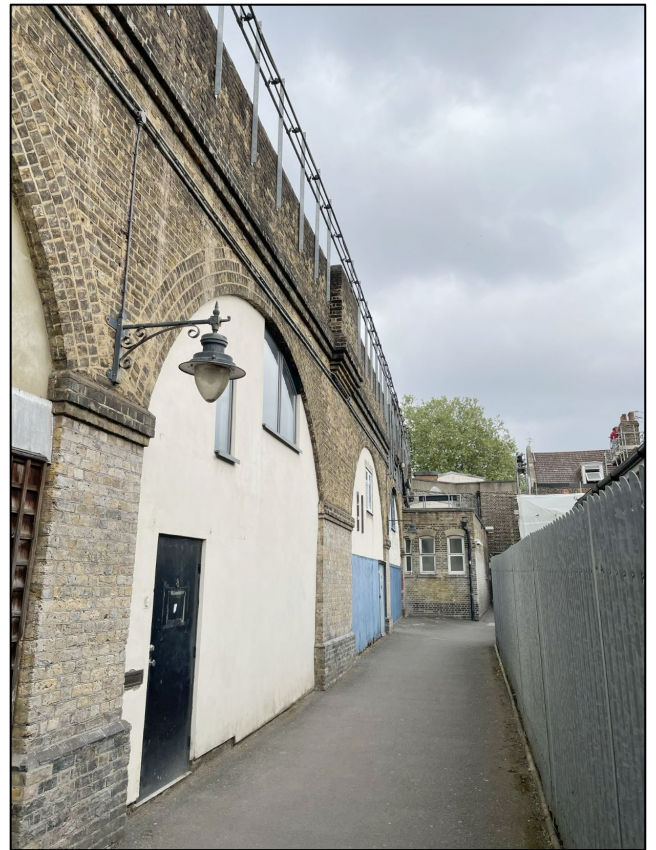
D76D viaduct and Wilson Walk.
