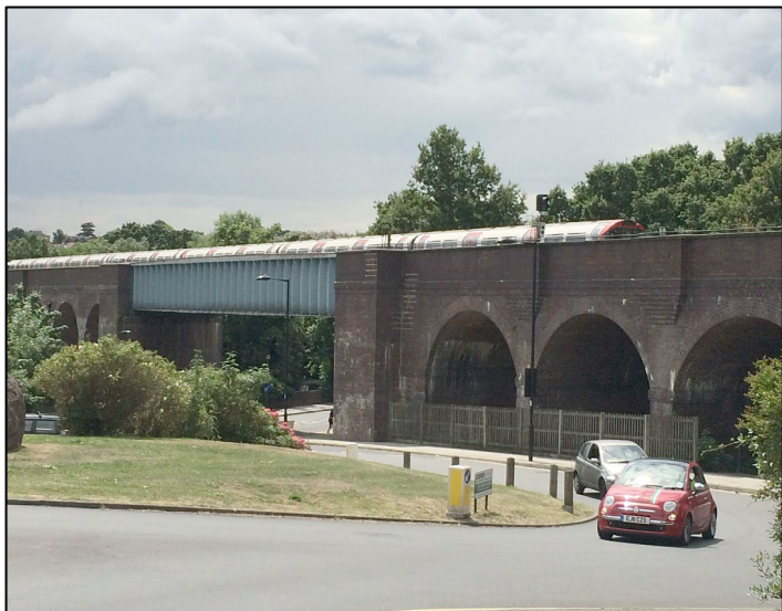
Short viaduct between Waterfall Road and Hampden Way.
