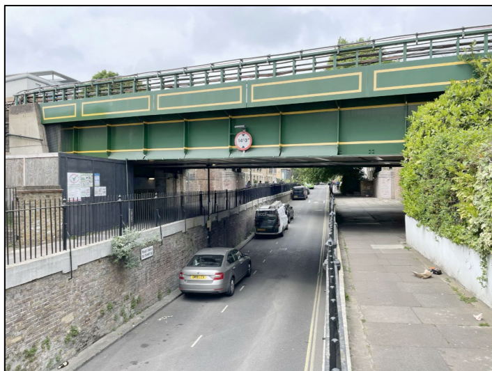
Above: D83 Cambridge Grove (south side) Below: D84, close up.
