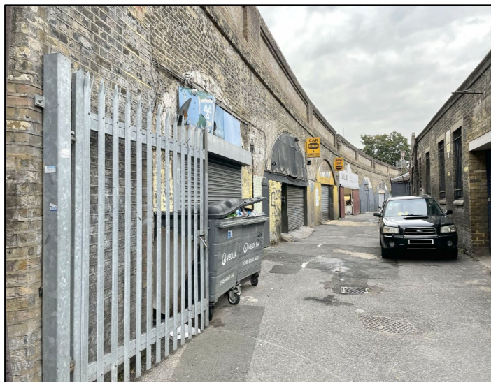
D93E Viaduct north of Hurlingham Road.
